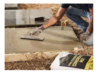
Concrete slabs are fundamental elements in modern construction, serving as the base for floors, patios, driveways, and more. A successful concrete slab depends on multiple factors, but one of the most critical is the <u>Mix for concrete slab</u> itself. Choosing the right mix ensures durability, strength, and resistance to cracking and environmental conditions.
